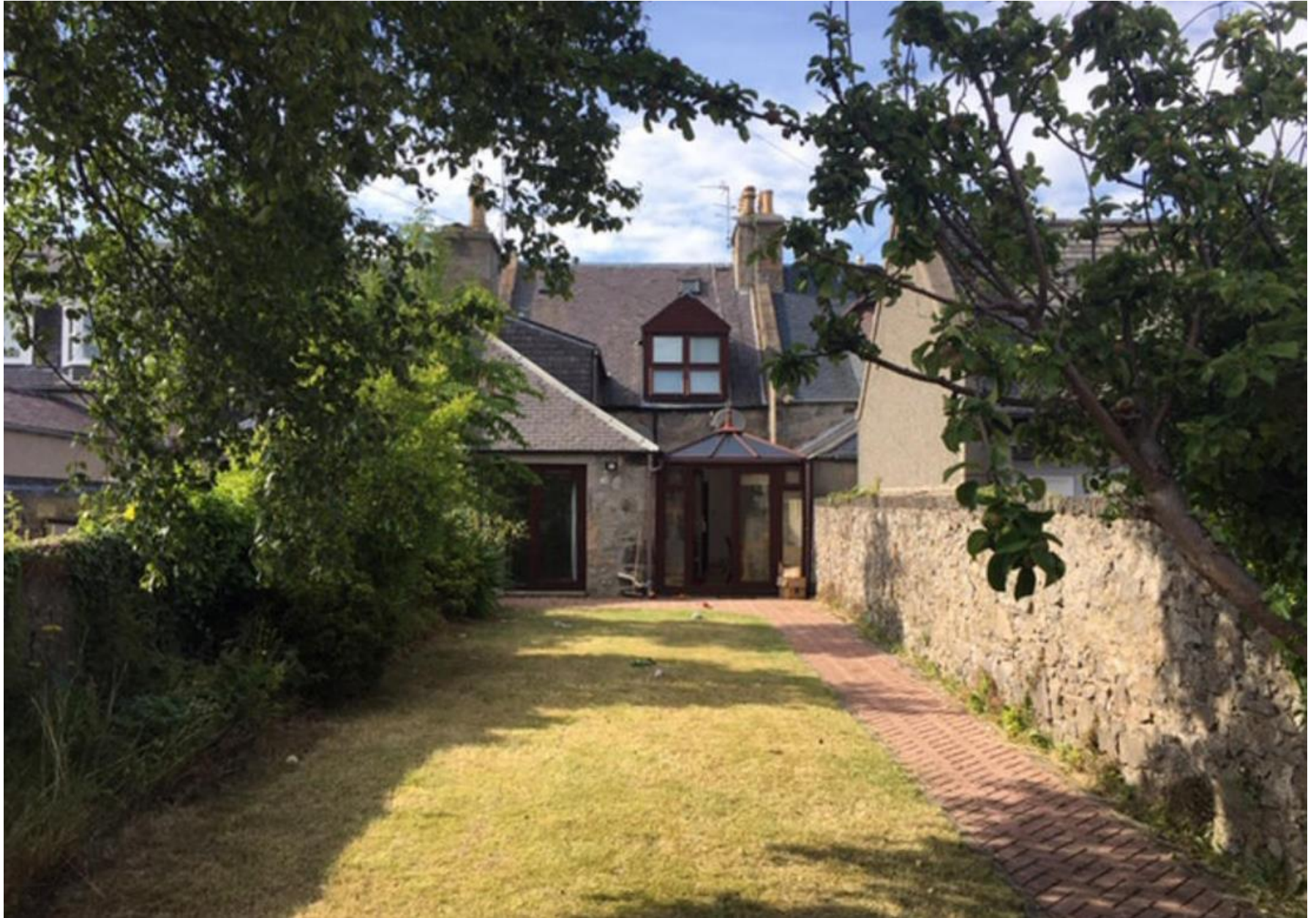
Photo: Rear Elevation
